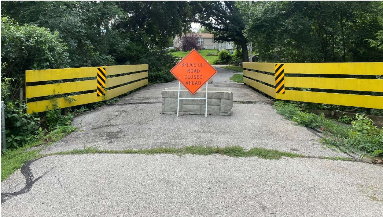
Looking south on Johnson Road at bridge (photo taken 8/14/2023)
