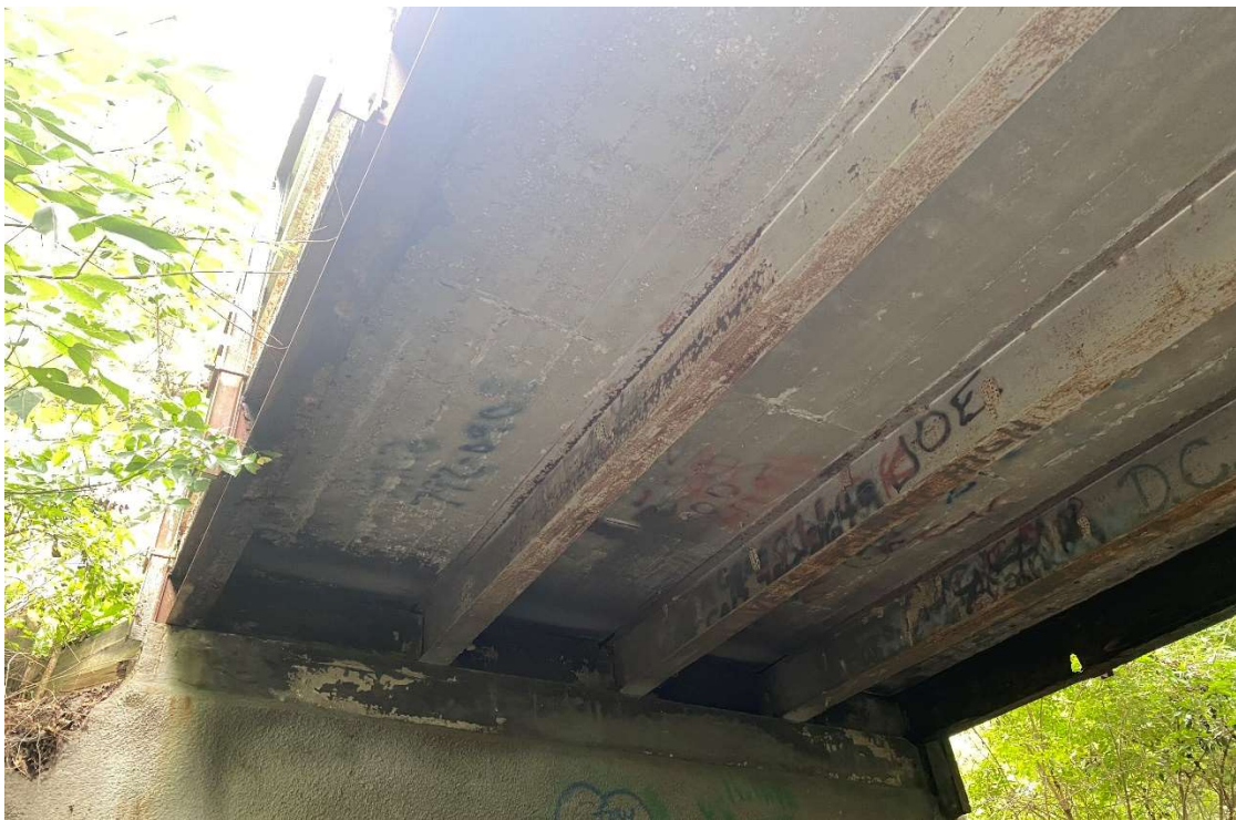
Looking underneath Johnson Road bridge (photo taken 8/14/2023)
