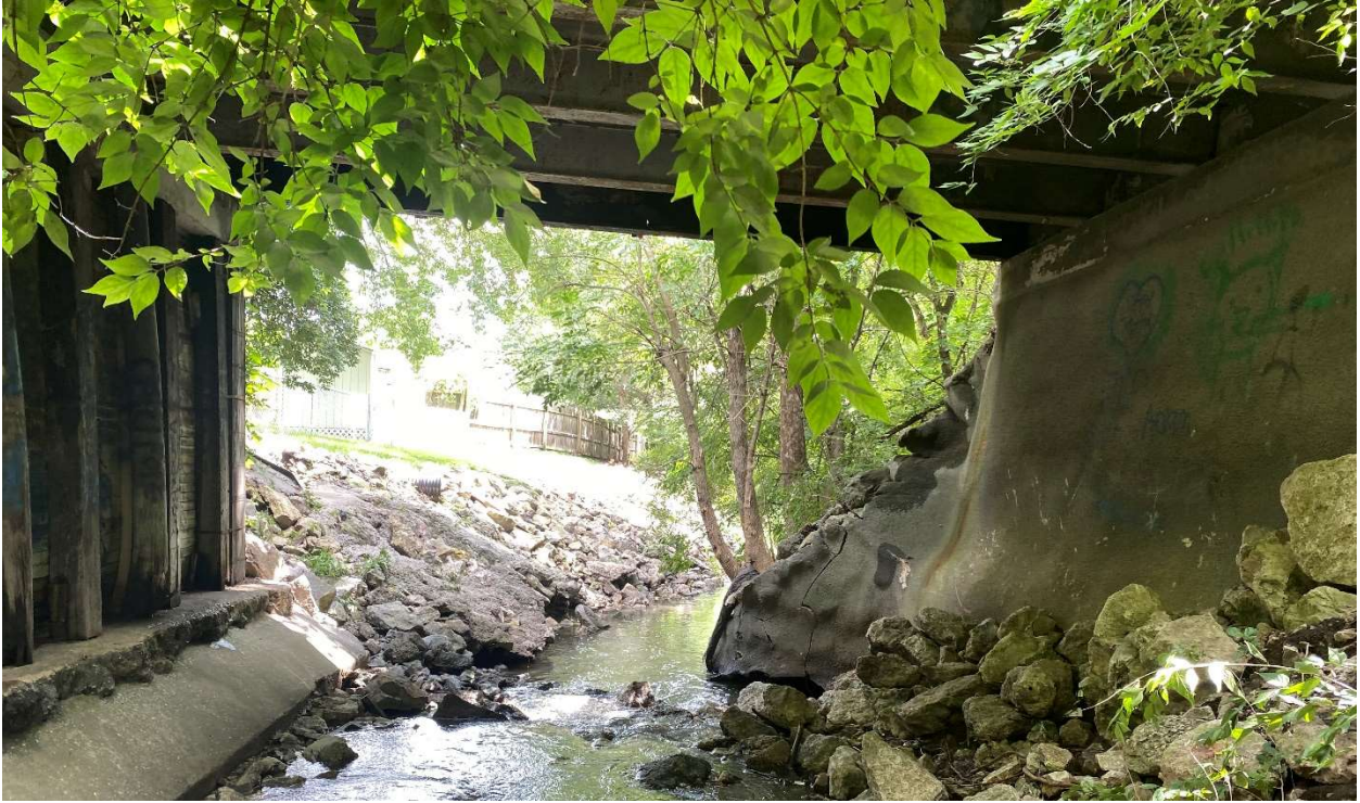
Looking underneath Johnson Road bridge (photo taken 8/14/2023)
