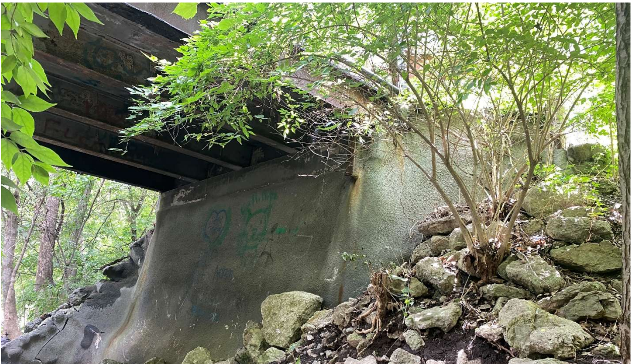
Looking underneath Johnson Road bridge (photo taken 8/14/2023)
