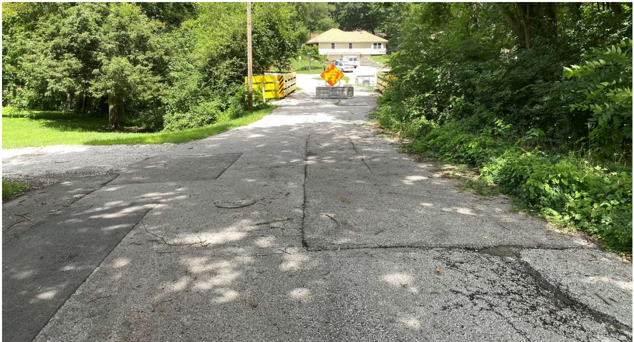
Looking north on Johnson Road at bridge (photo taken 8/14/2023)
