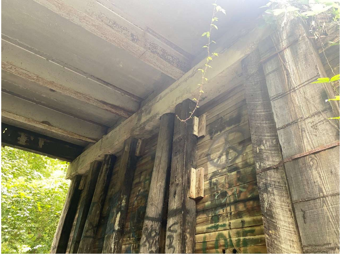
Looking underneath Johnson Road bridge (photo taken 8/14/2023)
