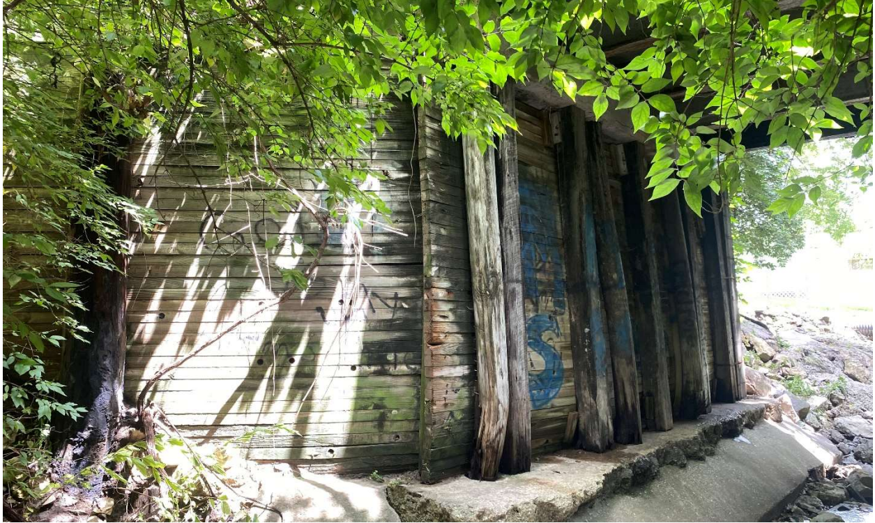
Looking underneath Johnson Road bridge (photo taken 8/14/2023)
